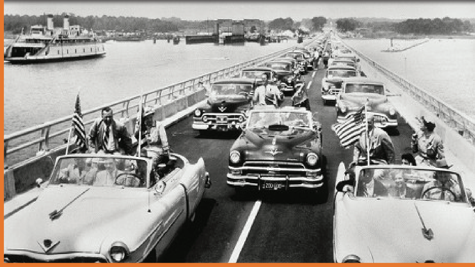
1952 - First Span (Two Lanes) Opens
