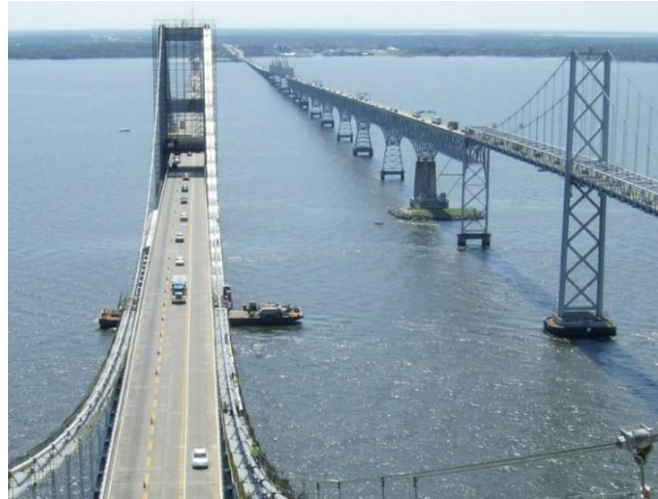
Figure 4: Existing Bay Bridge spans, looking east
