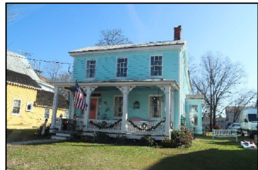
Figure 6-22: Turner House (Dr. J. E. H. Lewis House). Image Credit: RK&K, 2022.
