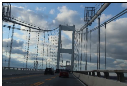
Figure 6-2: William Preston Lane, Jr. Memorial Bridge, Eastbound. Image Credit: RK&K, 2022.
