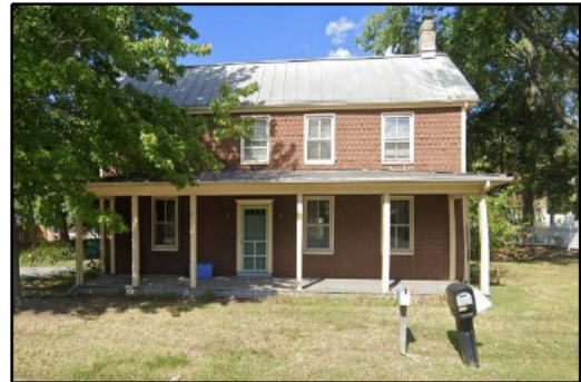
Figure 6-18: Gillis House. Image Credit: Google Street View, 09/2022.
