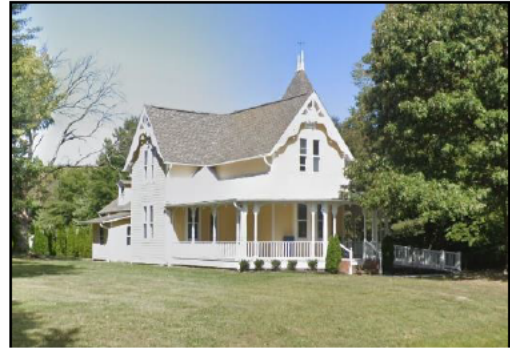
Figure 6-12: John Benton House. Image Credit: Google Street View, 09/2022.
